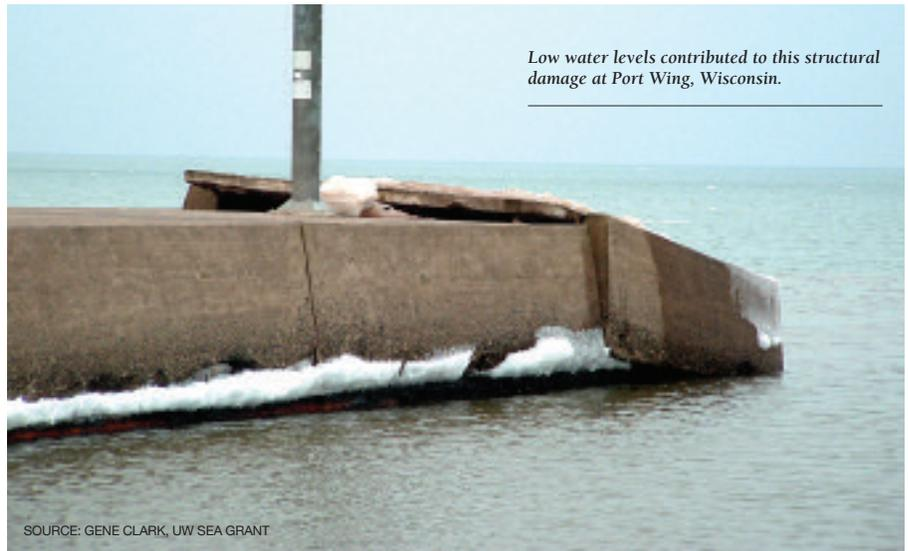
Low water levels contributed to this structural damage at Port Wing, Wisconsin.
